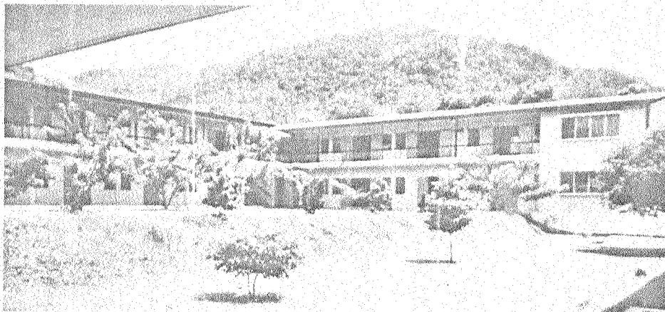
Malaysia's Federation School for the Deaf is housed in this new building—a monument to the patience and fortitude of the school's administration. The building was first planned in 1956, ground was broken 10 years later but not until 1969 did classes first meet in it. (This view shows a portion of classroom and dormitory buildings; the entire complex is too large to be photographed in a single view.)
